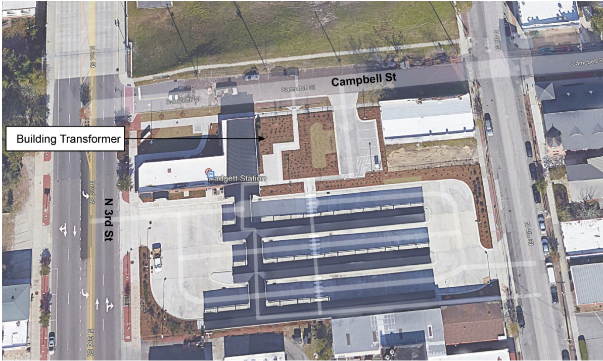
Figure 6. Padgett Station Aerial View
