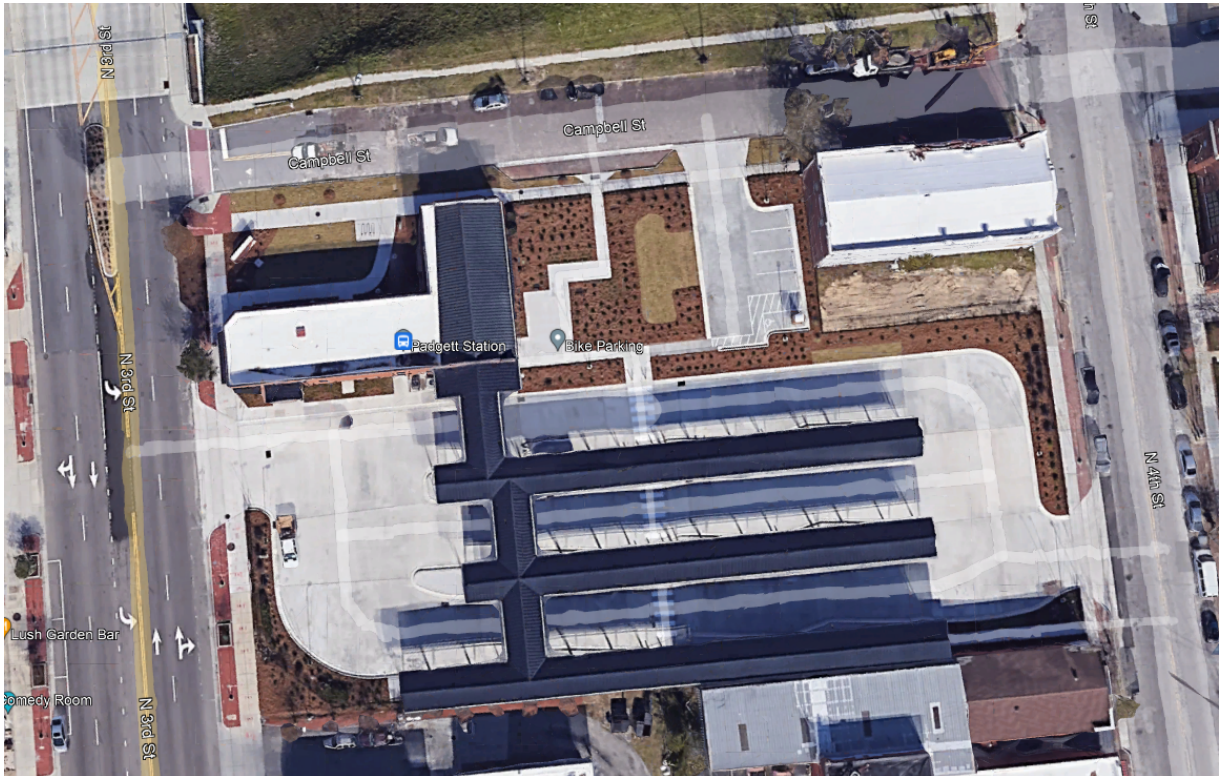
Figure 23. Padgett Station Aerial View
