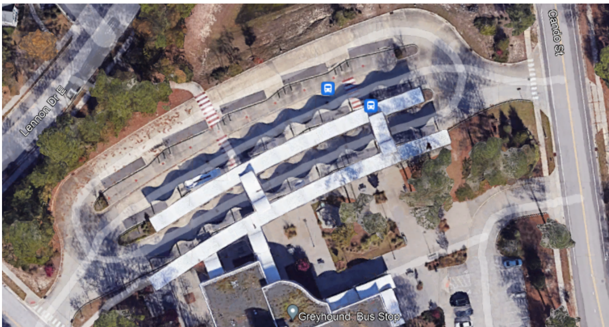
Figure 22. Forden Station Aerial View
