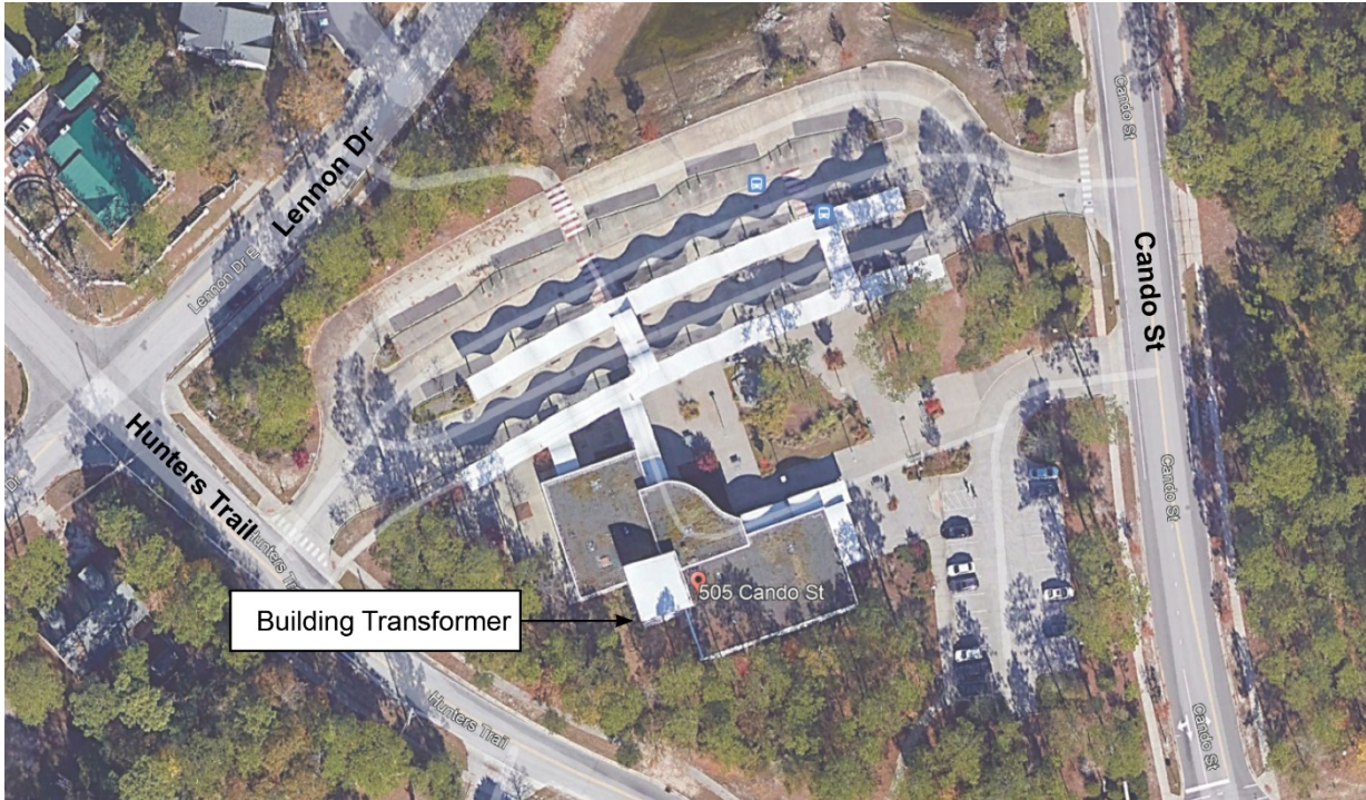
Figure 5. Forden Station Aerial View
